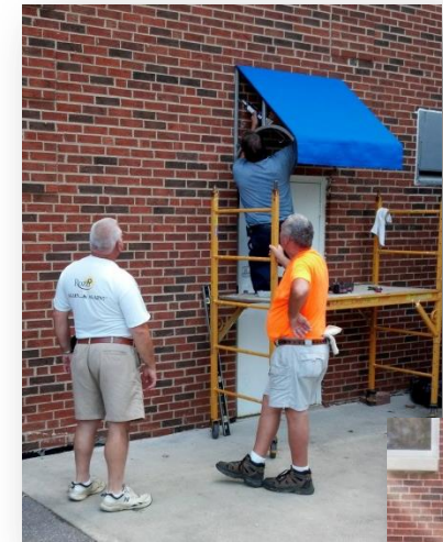
New Awnings Installed
